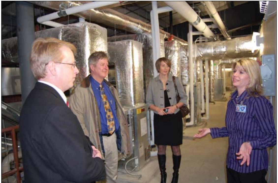
Bullitt County Schools Energy Manager Andrea Rock, right, shows visitors some of Roby Elementary School’s cost-cutting design functions, including geothermal heating and cooling and a state-of-the-art air filtration system. Gov. Steve Beshear used Roby Elementary to announce the Energy Manager grant partnership among the state, U of L and KSBA.
